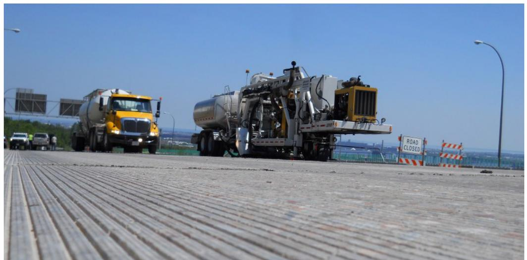
To groove a pavement surface, machines equipped with circular diamond-tipped saw blades are used to cut grooves into the surface. The blades are mounted and spaced on a horizontal shaft and are cooled constantly by water pumped from a tanker, which is recovered by an on-board vacuum system.
