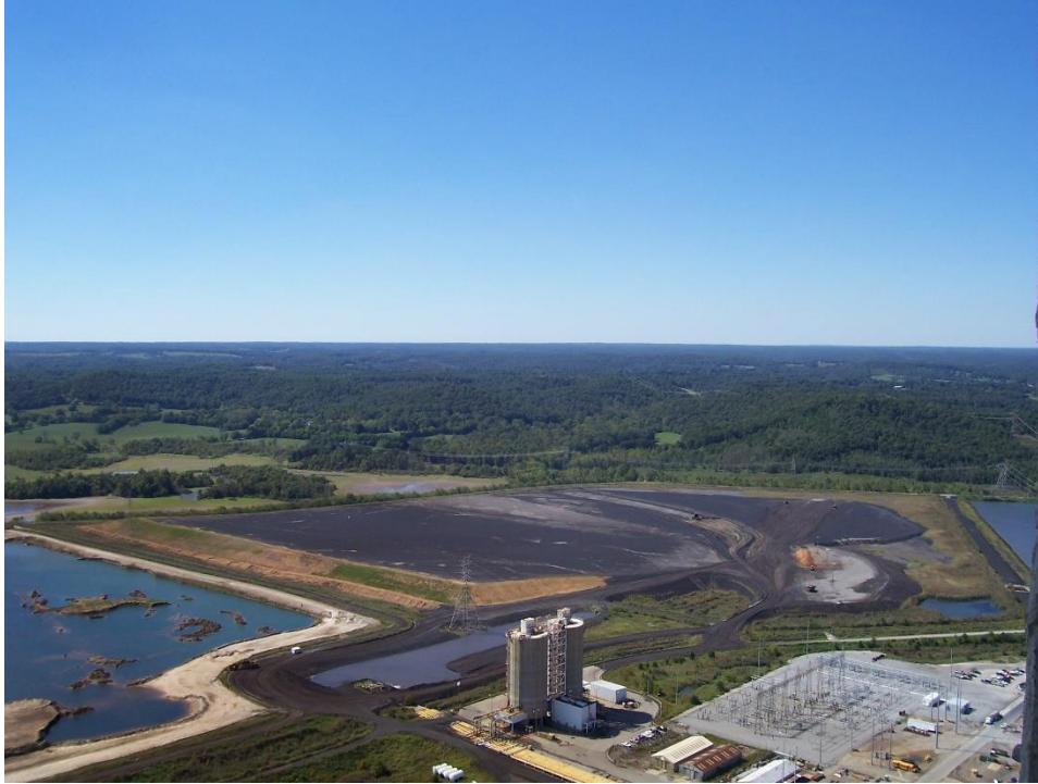
Figure 3.18-3. Aerial view towards the southwest of CUF Reservation and surrounding area showing part of the switchyard, silos, CCR, and wastewater management facilities
